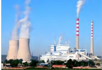
Self-supporting Power Plant
